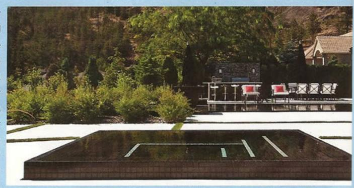
slowly raising from the deck," Brown says. "Everyone does a double-take [before they realize it's a spa]." That attention to detail goes below deck as well. Even though the spa appears to be separate from the pool, the half-inch slot surrounding the vessel actually flows directly into the pool's surge tank, so the entire body of water is cared for in one system.
