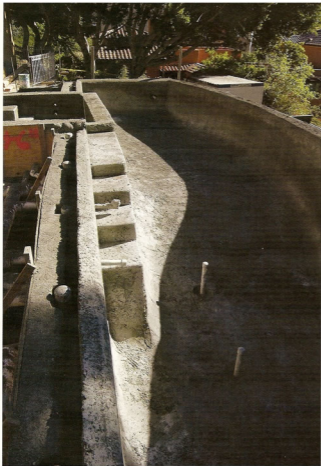
The completed shotcrete shell is then ready for waterproofing and veneers
