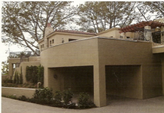
This view reflects the support structure and integrated upper pool wall at completion. The deep end of the pool is located behind the double doors and the shallow end rests on the carport
