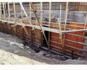
The construction processes followed with poured in place concrete allow a measure of precision that is much harder to come by when using pneumatically applied material – a wanderful advantage when it comes to executing rectilinear designs and all-tile finishes because the walls are so amazingly clean when the forms are pulled.
