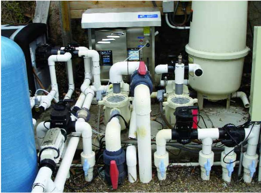
The use of VFD pumps simplified my equipment pad by reducing the number of pumps from three to two – a small saving in space but a substantial one with my utility bills. In profile, the VFD models aren't much different in appearance from conventional pumps, but they more than distinguish themselves when it comes to performance.
