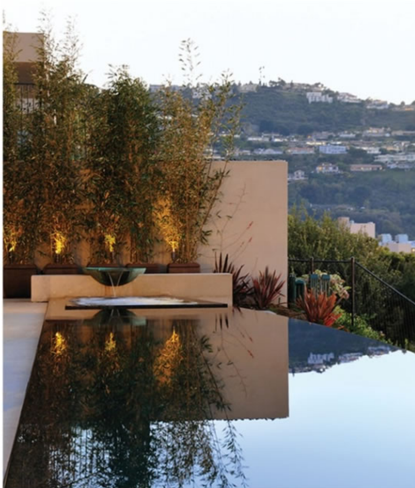
This pool, with a 160-foot edge, has no turbulence. The spa was used to diffuse the potential turbulence. Designer: Bruce Rudd, Island Architects / Skip Phillips; Builder: Skip Phillips
