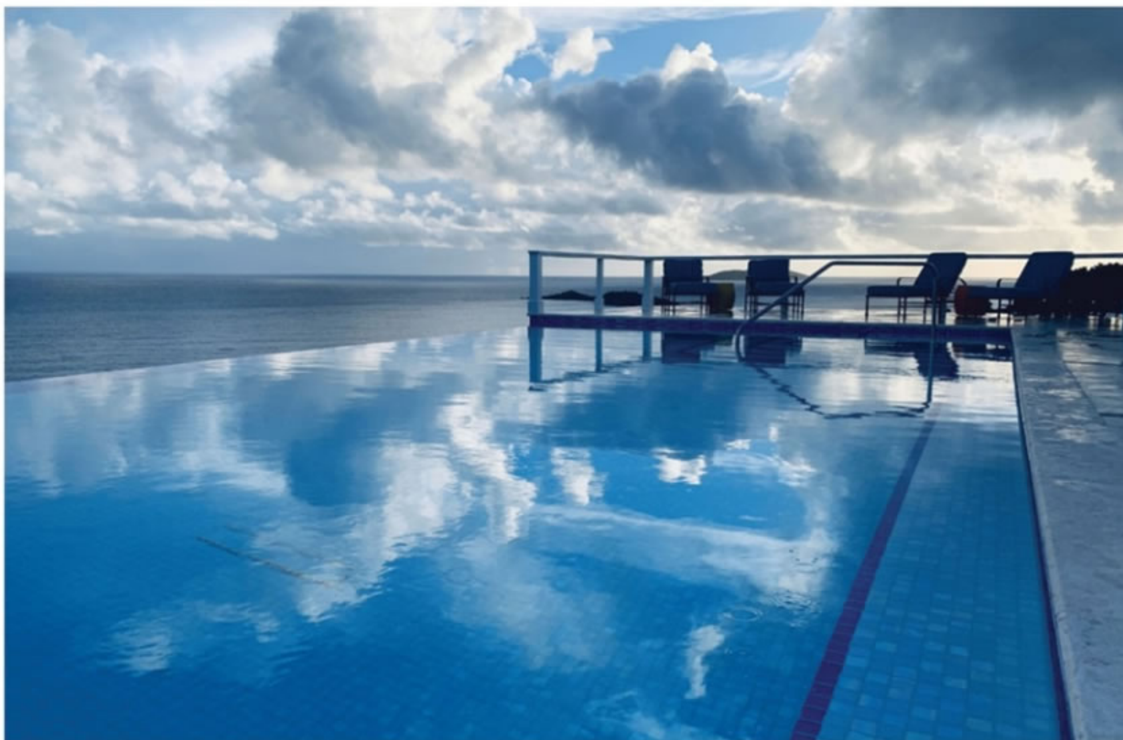
This vanishing-edge pool was completely rethought during a renovation, both mechanically and cosmetically. Designer: Skip Phillips; Builder: Mike Fuller, Poolworks
