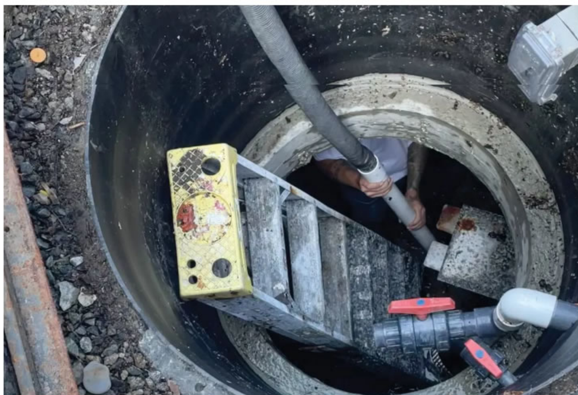
Vacuuming is one of the best cleaning methods if the surge tank is accessible. Photo: Strange Pool & Spa
